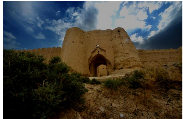
Figure 6: Architecture of Rostam Castel (photograph by Kavosh).
