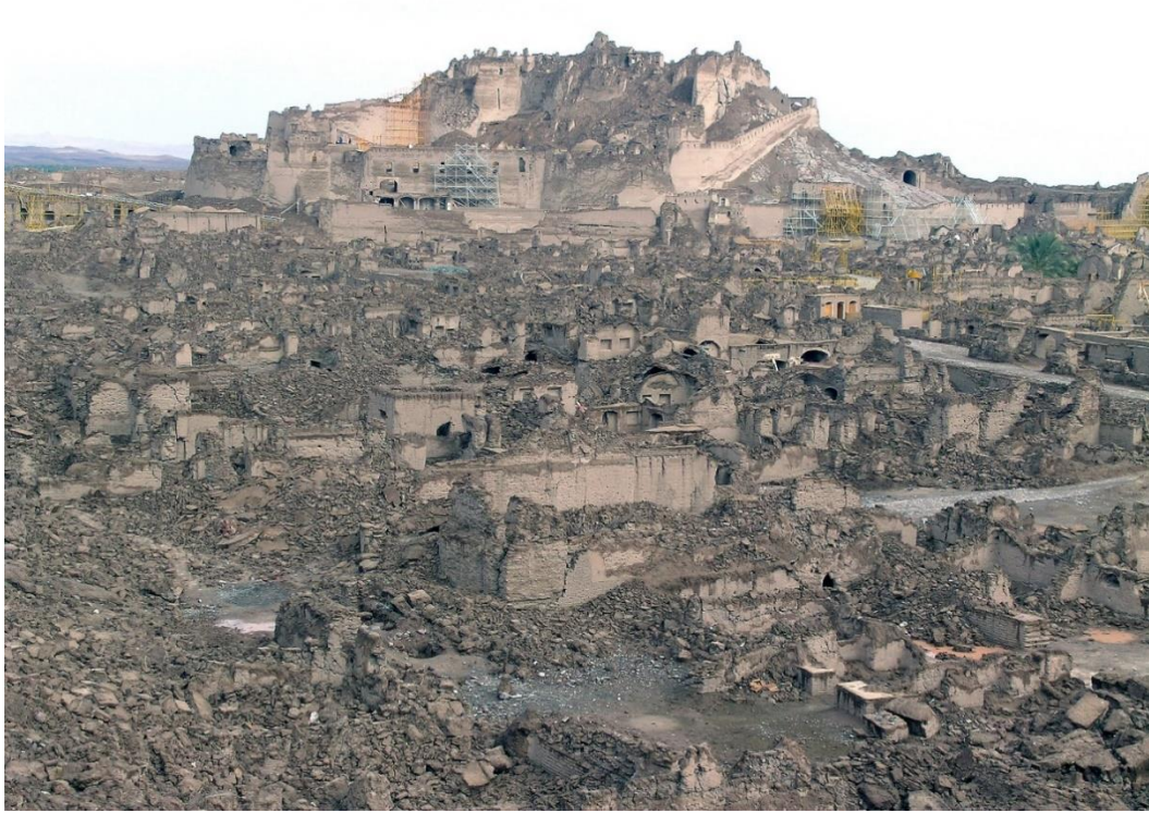
Figure 1. Arg-e Bam after the earthquake.
