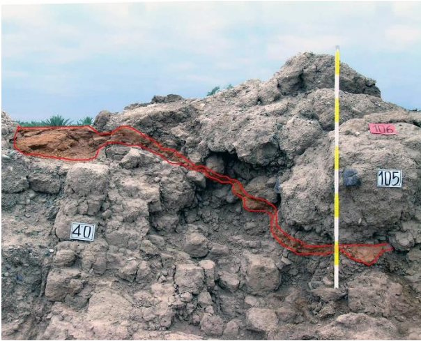
Figure 13. Negative interface (US 106) from pre-2003 seismic event documented near the southern walls standing on the eastern side of the ancient tower.
