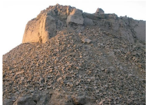
Figure 3. The tower after the calamity.
