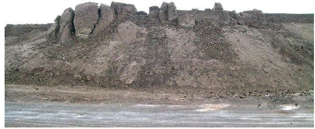
Figure 29. West side of tower n° 46 ( Shotor Galu ) before excavation.
