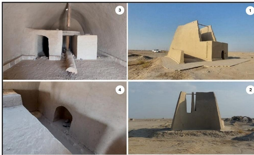
Figure 5: The windmill (Asbad) No. 2 of Hozdar (Small Asbad) (authors, 2023)
