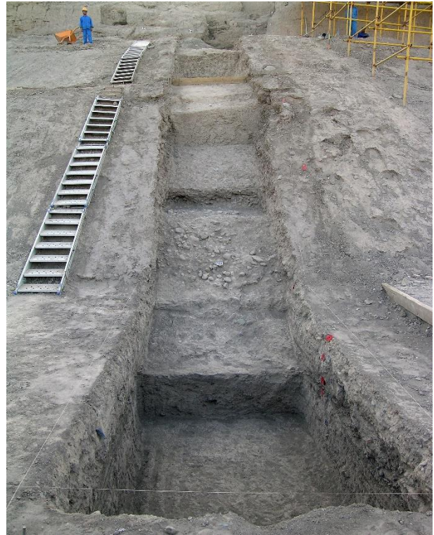
Figure 19. Excavation of the city wall rampart.
