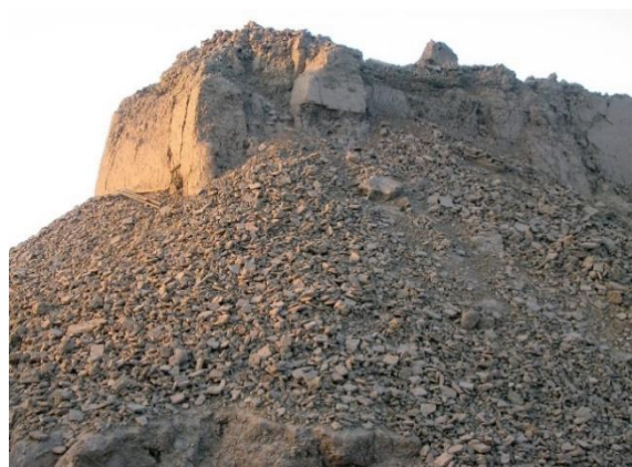
Figure 3. The tower after the calamity.
