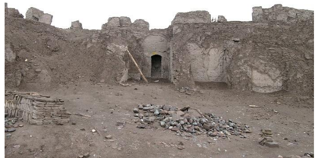
Figure 30. East side of the tower seen from the inner city before excavation.
