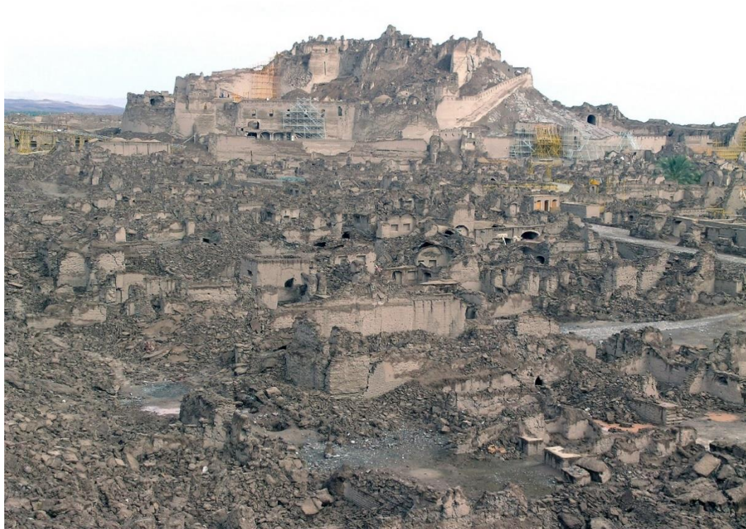
Figure 1. Arg-e Bam after the earthquake.
