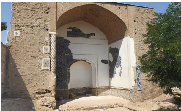
Figure 2. Overview of the Remaining Porch of the Qobbeh Sabz Building (Authors).
