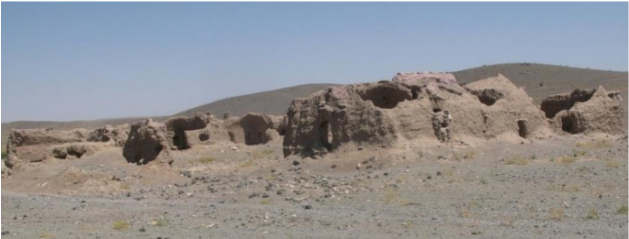
Figure 10. West side of Koohakrud Caravanserai (by Authors, 2019).
