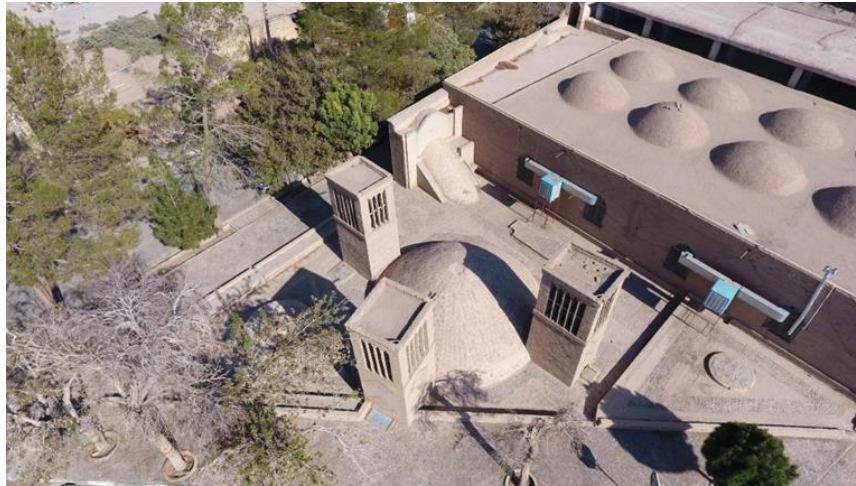
Figure 18: Aerial image of the Amin Shahr Reservoir.
